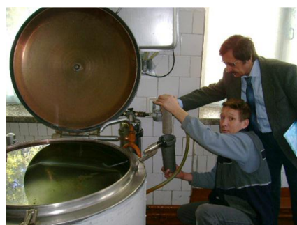
Picture 3. Water-filter installation in Mailuu-suu school n 5 kitchen
