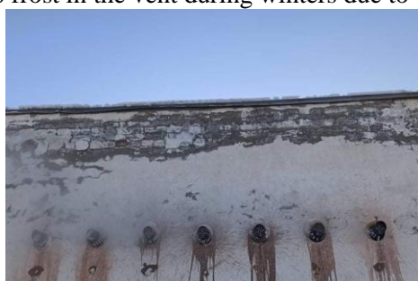
Fig.1. Frosting over of the gas boiler vent
