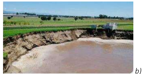
Fig. 23. Photographs of the site with sinkhole in Mexico.
